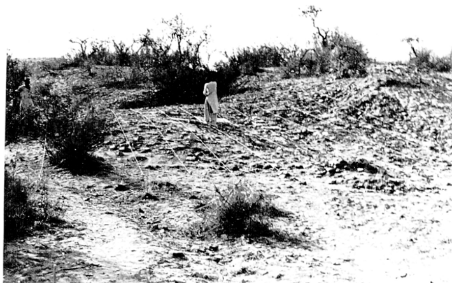
a) Moenjodaro, AA. 47. View of the site from east.
